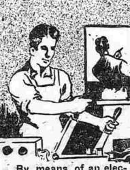
By means of an electric current a shell . of copper is laid on the wax sheet and this takes the lines of the original
